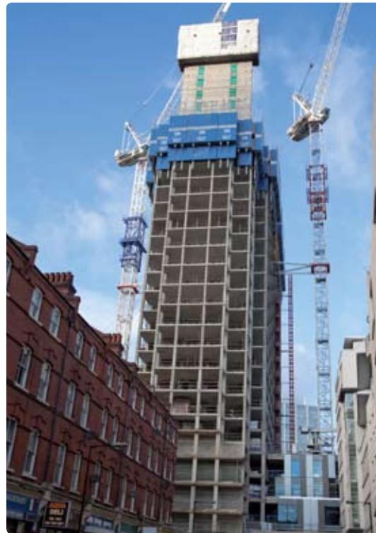
Figures 4 and 5: Work on the core started in March 2008 and completed, at floor 34, in December 2008.
